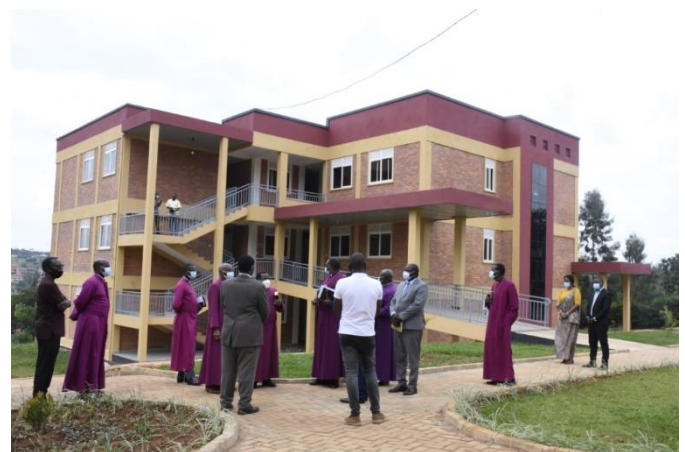
Second brand new dormitory building
