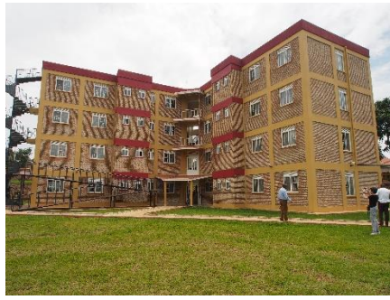
KATC Dormitory – finished!
