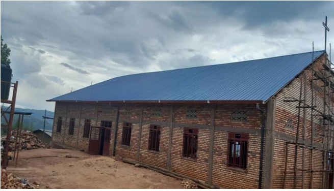
Building of new parish Church Nkorwe
